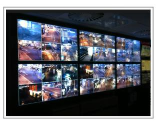
There are two (2) other additional benefits gained from this type of wall. The amount of space required for a display wall of this type is much less, so some floor space within the control room will be realised. The other significant benefit from LCD monitors is the much reduced power consumption compared to standard CRT<sup>2</sup> monitors and subsequently the amount of heat produced by these monitors will be much less.
